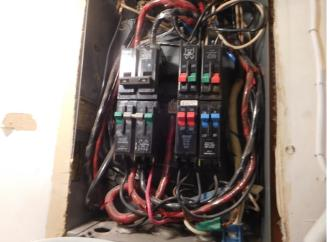
The GFCI outlets that were tested functioned properly. Ground Fault Circuit Interrupter (GFCI) electrical outlets and breakers are a significant safety improvement and are required for bathrooms and kitchen counter top outlets, outside outlets to reduce potential electrical hazards in wet areas.
