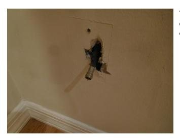
The missing cable cover in the living room for the cable that is stuck in the wall needs to have a new cover installed.
