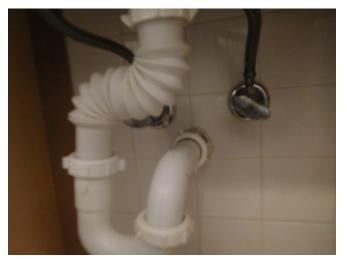
The flex drain under the bathroom sink is not a recommended drain connection because it can accumulate soap scrum in the grooves and start to smell over time
